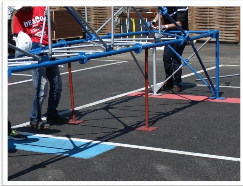
Figure #1: Temporary Support Members (brown painted elements.)
